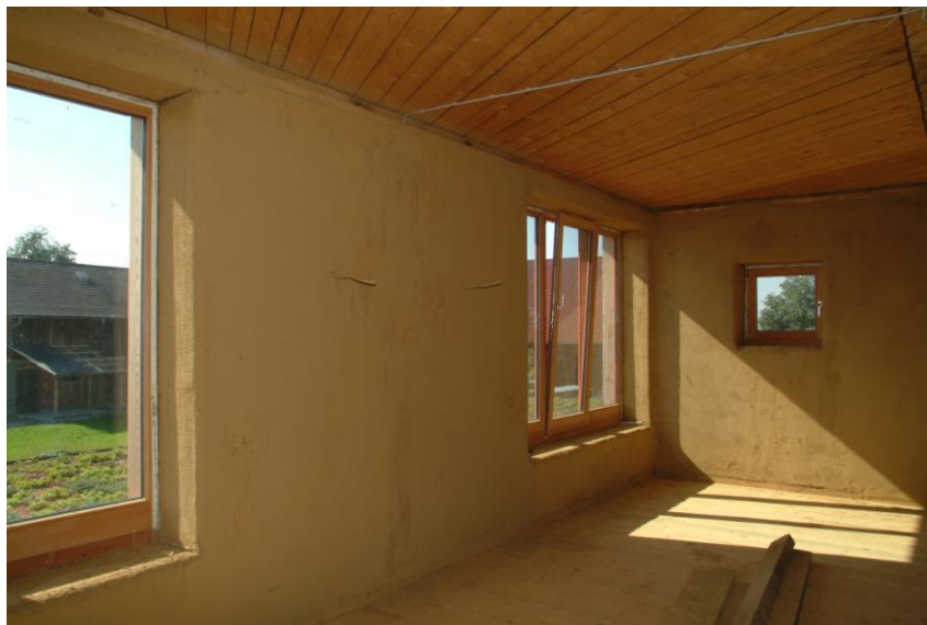
Figure 27 .Earth plaster of straw bale building
